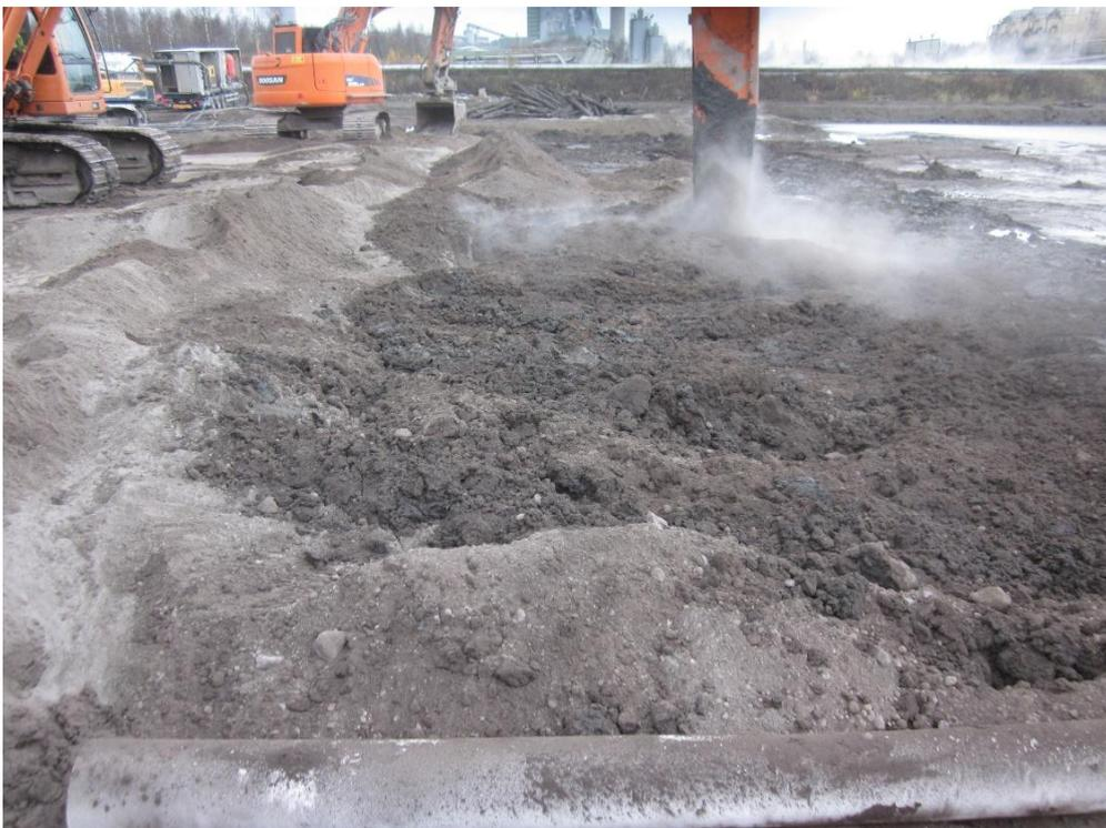
Figure 6. Mass stabilization with high (350 kg/m<sup>3</sup>) binder amounts
